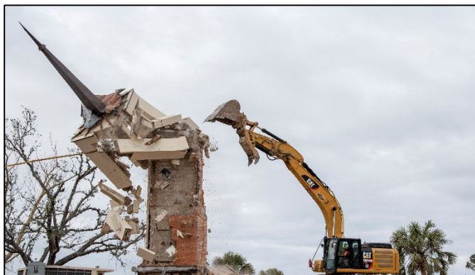
Demolish 247 of 484 Facilities
